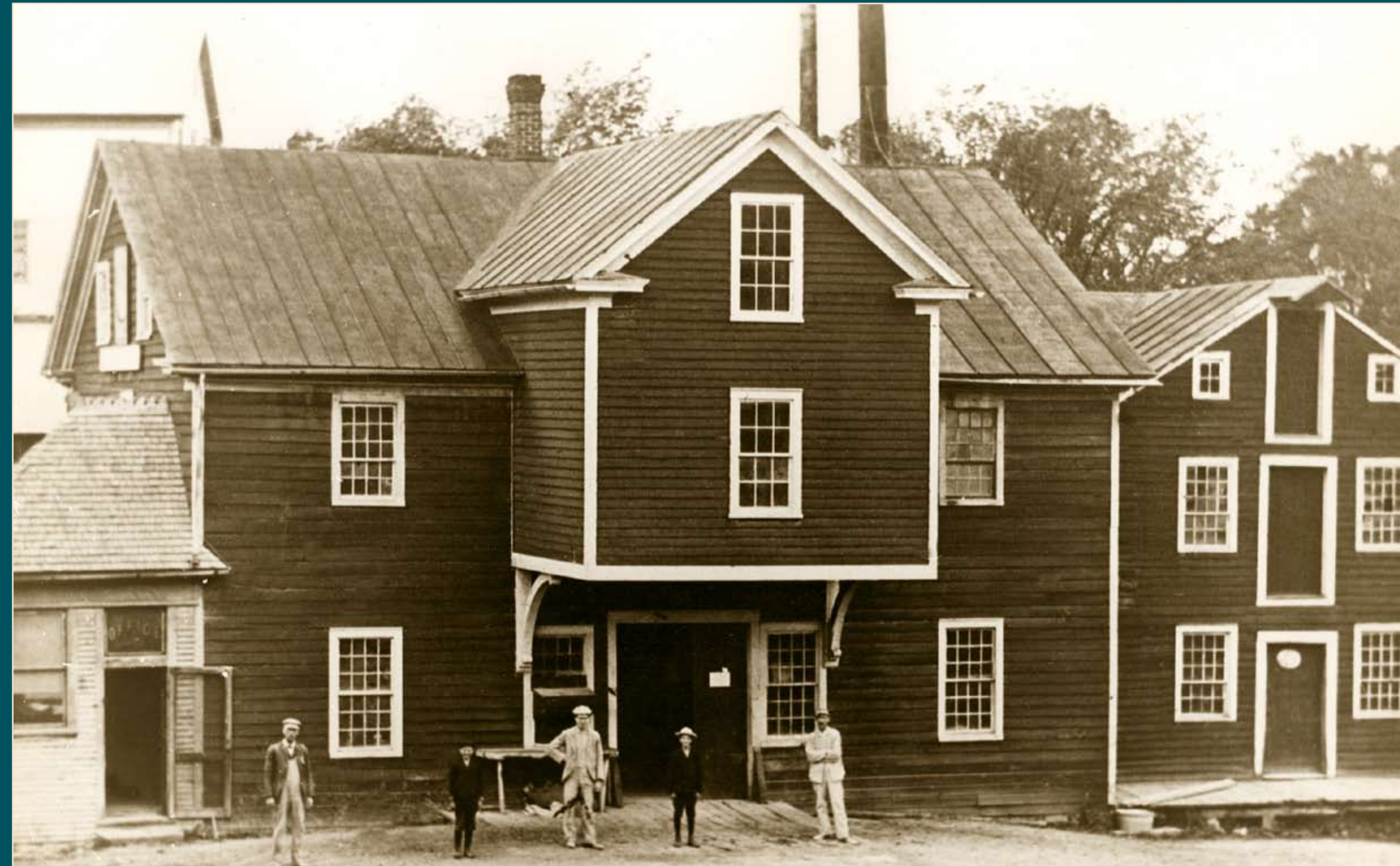
The gristmill, where farmers would bring a wide variety of grains, including buckwheat, oats and corn, to be ground into flour or animal feed. Milling was a three-story process. The grain was lifted in sacks onto the top floor of the mill by hoist. The sacks were then emptied into bins, which fed the grain down through a hopper to the millstones on the floor below. The grain then flowed through a sloping trough into a hole in the center of the top stone. The milled grain (flour) was collected as it emerged through the grooves in the bottom stone from the outer rim of the stones and was fed down a chute to be collected in sacks on the ground floor. Photo courtesy of the Town of Peru Historian’s Collection.
