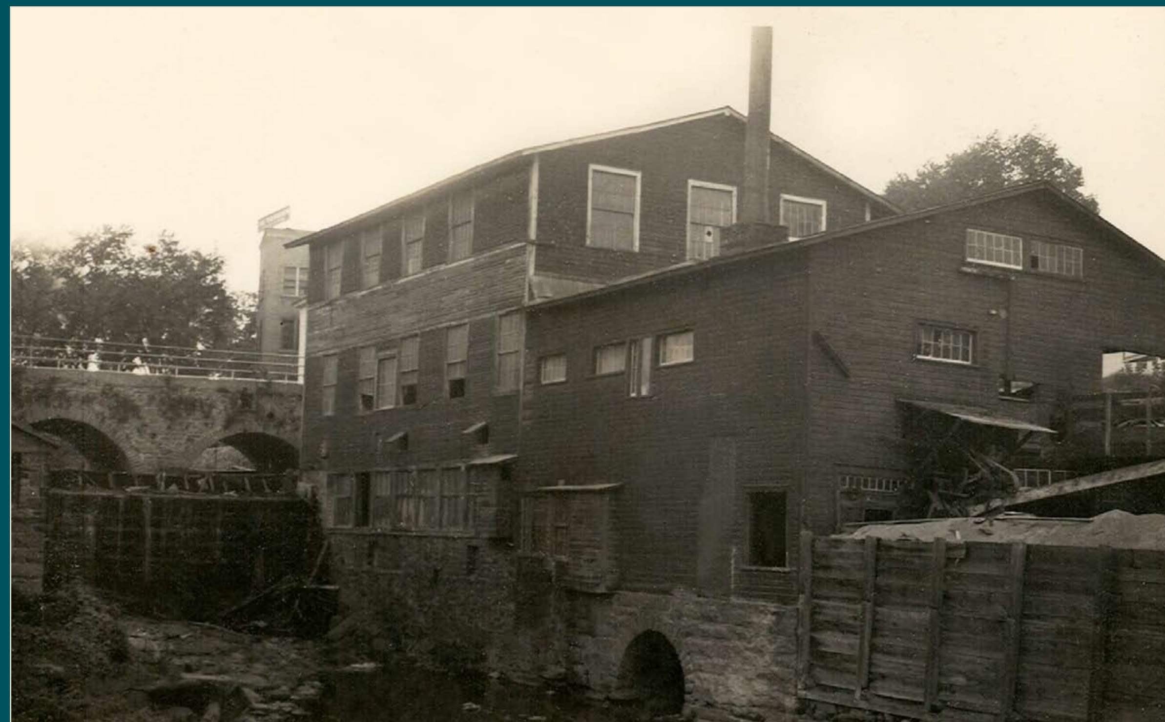
The sawmill, as part of A Masons and Sons Lumber Mill, c. 1900. Please note the stone arch on the river that’s still visible today, where water that had carried the logs to the mill flowed back into the river. Photo courtesy of the Town of Peru Historian’s Collection.
